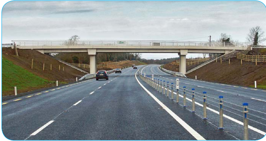
Construction of new roads.
