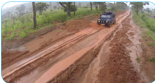
Poor road network.
